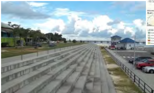
COE Seawall, Bay St. Louis, MS
